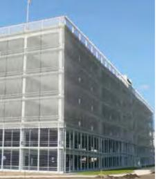
Facade cladding of a parking garage with the HAVER Architectural Mesh DOGLA-TRIO.
