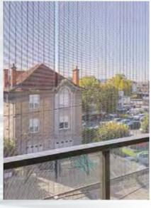
The open geometry of the architectural wire mesh preserves the view on the outside wor-Id. Facade cladding MULTI-BARRETTE 8123, Brive-la-Gaillarde, France.
