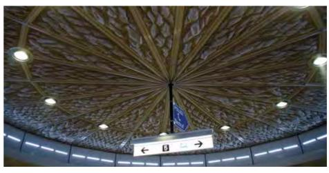
Three-dimensional stainless-steel mesh for improving the space's acoustics. Cologne light railway, Germany, MONTANA.
