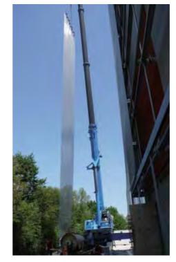
Large mesh elements are quick and easy to assemble. Once assembled, HAVER Architectural Mesh requires little to no maintenance.
