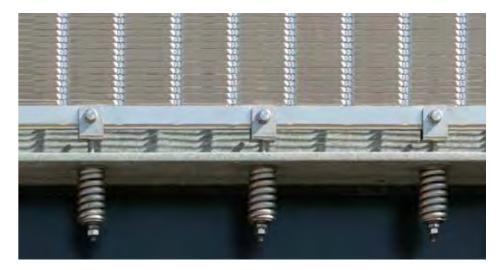
Mounting solution for wire mesh facades.
