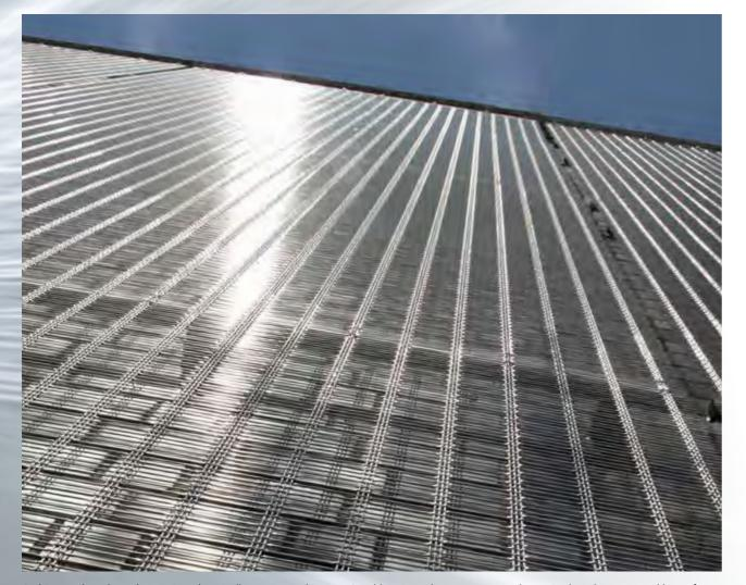
Architectural mesh can be tensioned vertically over several storeys. Load-bearing substructures are only required on the upper and lower face. Facade cladding DOGLA-TRIO 1032, Germany.
