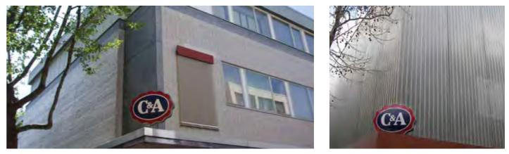
The semi-transparent stainless-steel mesh LARGO-NOVA 2017 encloses the existing building and ensures natural lighting. C&A Eco Store, Mainz, Germany.
