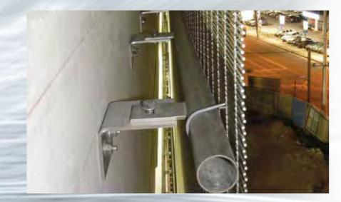
Intermediate mounting: round tube and wire connectors.
